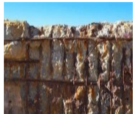
Fig 44:- Effect of corrosion in reinforcement
